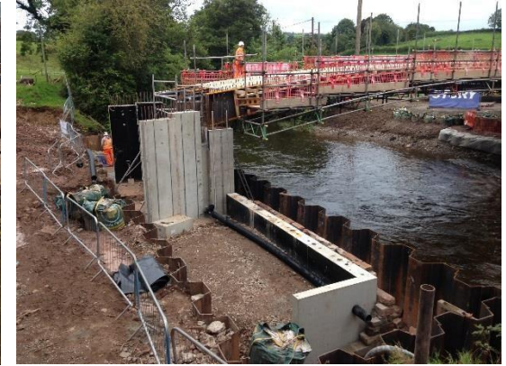
View from the East Abutment
