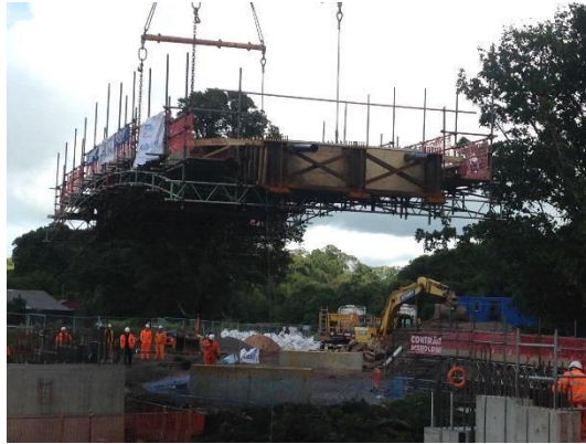
Lifting the deck into position John Slee
