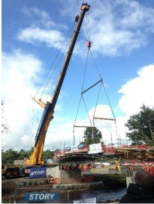
Lifting the deck into position John Slee
